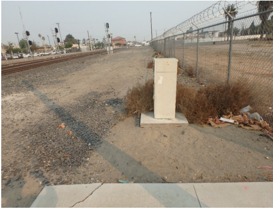
Figure 3.6-5: Disturbed coarse silty sand by electrical box with some exposed disturbed sediment along the tracks at East Main Street, view northwest.
