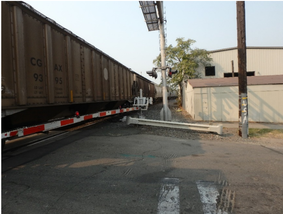
Figure 3.6-1: Narrow, unsafe right-of-way along the tracks near South Pilgrim Street, view southwest.
