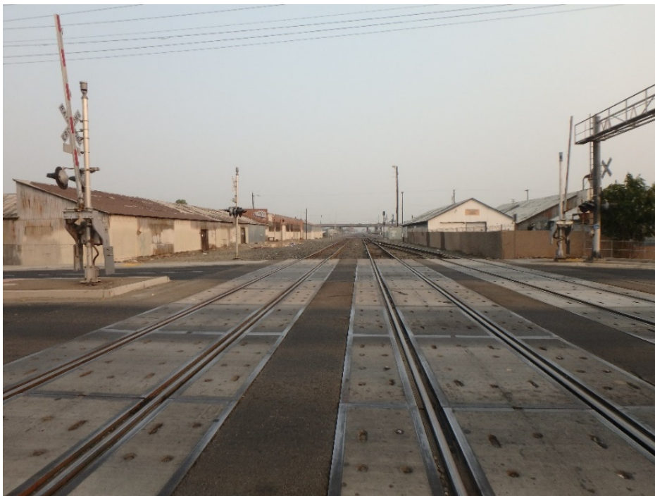
Figure 3.6-2: Typical disturbance along the right-of-way at East Hazelton Avenue, view northwest.
